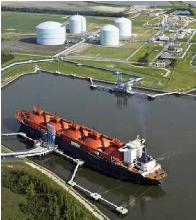
Insulated low pressure storage tanks for LNG
