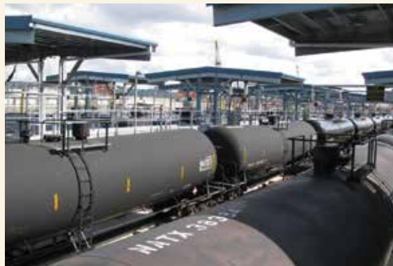
Rail loading facility.
