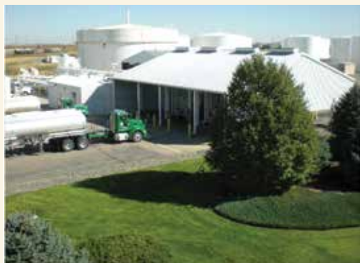
Truck loading facility.
